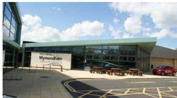
Wymondham Leisure Centre GMV5 Heat Recovery UK
