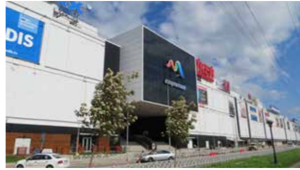
Sochi More-Mall Centrifugal Chiller Russia
